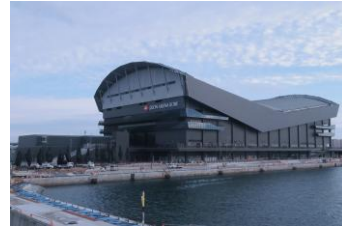
G LION ARENA KOBE (建設中)
